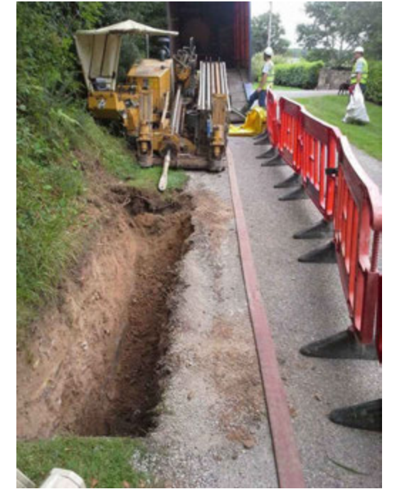
Image 2 : Typical Drilling Rig and Launch Pit
